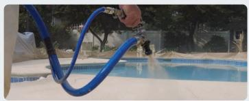
When spraying, it is preferable that Tuff Coat is at room temperature (or warmer) for easier spraying.
