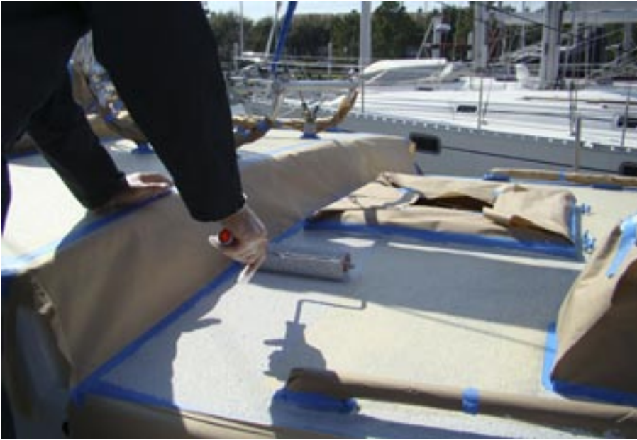
Chuck applies the first of the needed two coats of non-skid with a roller.
