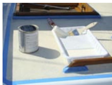
No special equipment is needed for the application, just a textured paint-roller cover and a small brush for areas the roller can't reach.
