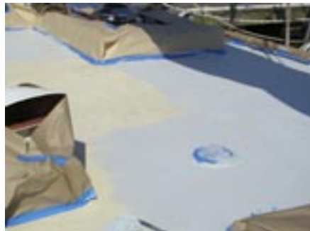
In areas the roller can't reach, the product can be dabbed on with a brush, above left. The first coat is applied in areas about a yard square to ensure it goes on evenly, above right.
