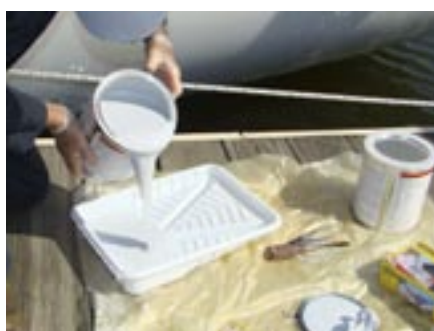
No special equipment is needed for the application, just a textured paint-roller cover and a small brush for areas the roller can't reach.
