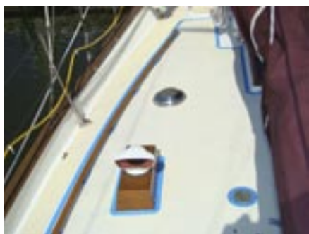
After removing from the deck whatever fittings they reasonably could, Chuck and Susan taped around what remained, above, then added masking paper as further protection, right.
