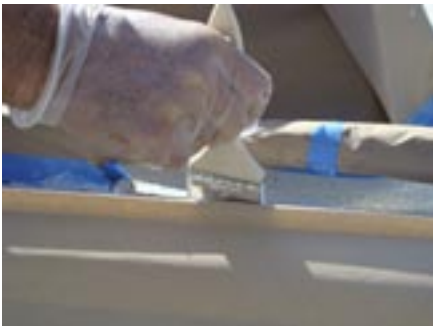
In areas the roller can't reach, the product can be dabbed on with a brush, above left. The first coat is applied in areas about a yard square to ensure it goes on evenly, above right.
